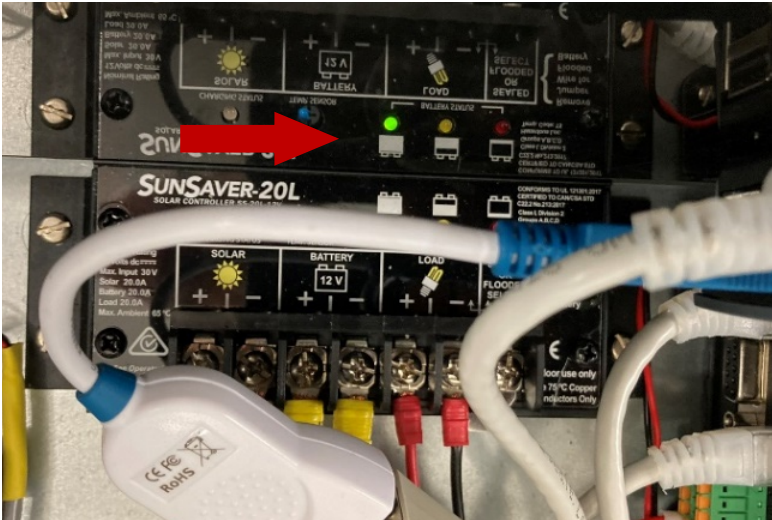
Figure 51. SunSaver LEDs showing battery status on the solar charge controller.
